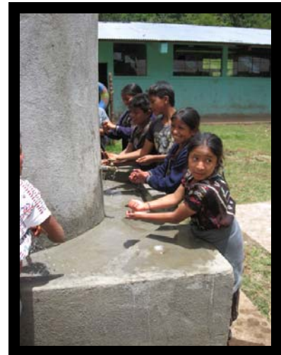
Students using the finished hand washing station
