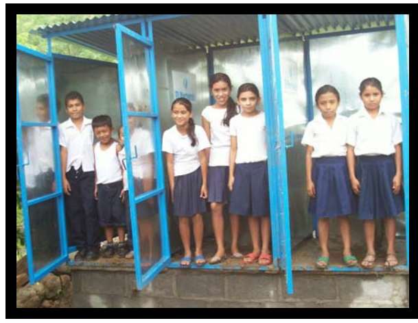
New school latrines at Rinconada School
