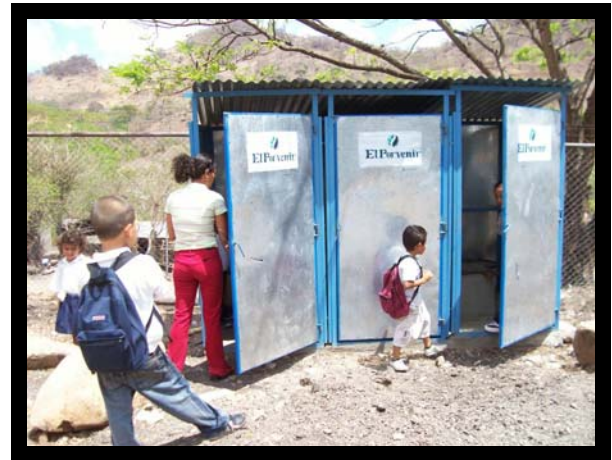
After: New latrines for students
