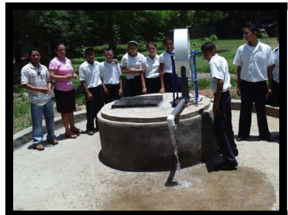
After: New rehabilitated well
