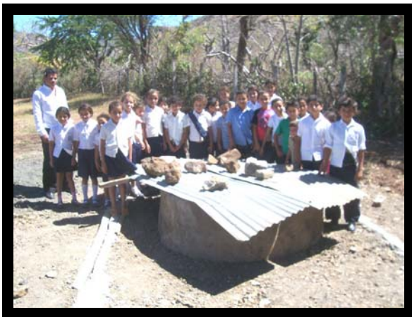
Before: Students in front of damaged well at La Uva School
