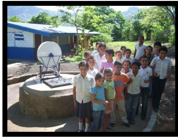
After: New rehabilitated well
